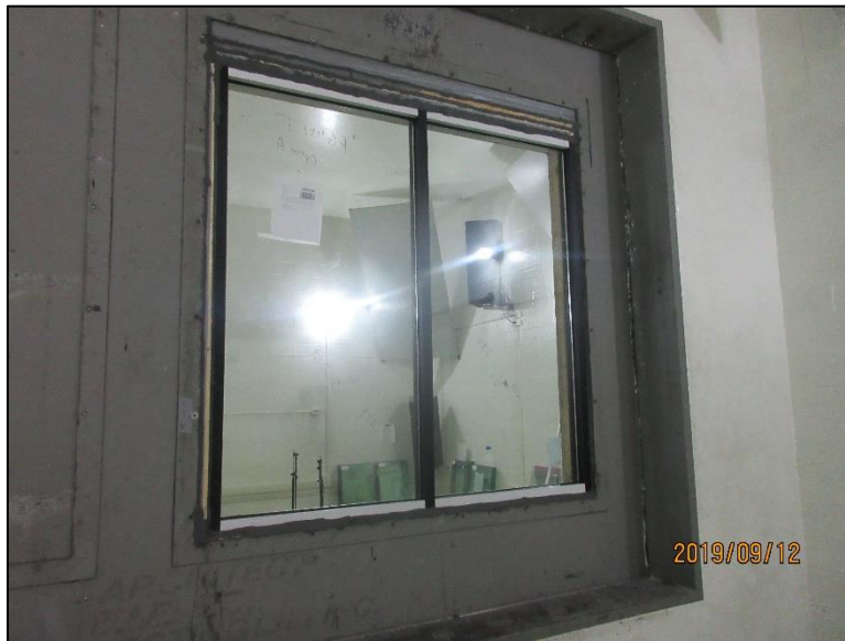
Photo No. 1 Receive Room View of Installed Test Specimen
